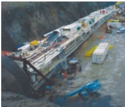
TBM Baustellenmontage Guadarrama Nord
