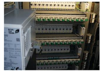
Eaton's SmartWire-DT intelligent wiring and communication system saved about 80 hours of labor to build the two switch cabinets for the two drilling vehicles – this time includes wiring, I/O testing and commissioning.
