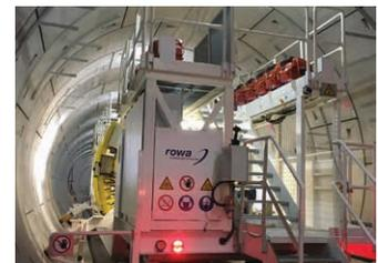
A perfect fit – the first drilling rig drills all the holes that will accommodate brackets for cabling, walkways and fire mains. The second machine focusses on the holes for the overhead electricity line, which will power the Crossrail trains.
